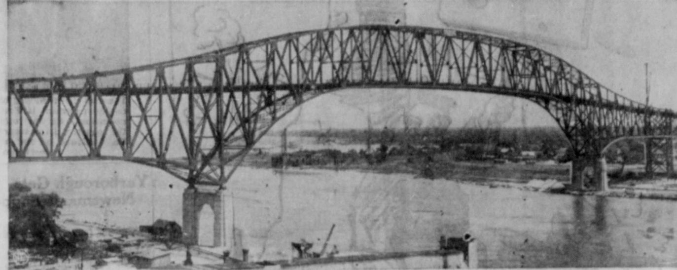
Another steel link binding the United States and Canada will be welded when President Roosevelt goes to Canada in mid-August to dedicate the Blue Water International Bridge pictured above. The bridge, 8000 feet long, and arching 152 feet above the waters of the St. Clair river, connects Port Huron, Mich., with Sarnia, Ont. It cost almost $2,000,000, and commands an impressive view of the junction of Lake Huron with the St. Clair river, a point where teeming lake traffic funnels through the narrow channel. The American and Canadian governments built the respective approaches, and an international commission built the center span. The bridge opens a new fast route between Chicago and Montreal.
