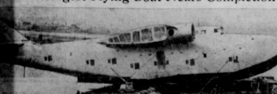
A side view of the new South Seas clipper which, when completed, will be the world's largest flying boat. Built in the Boeing aircraft factory at Seattle, Wash., the clipper will have a wing of 152 feet, and an overall length of 109 feet. It will weigh 42 1/2 tons when loaded, almost as much as the clippers now in use. First of six such ships to be constructed, the clipper will carry 72 passengers on daylight trips and 40 on overnight journeys.
