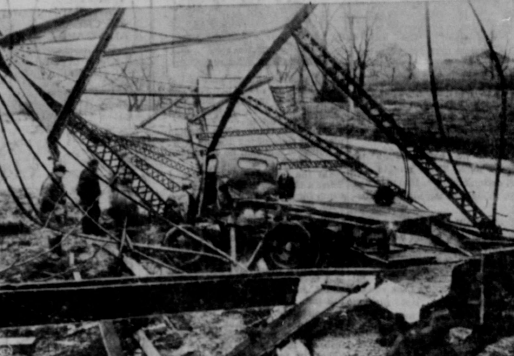
Frankfort's bridge—not Loadon's—has fallen down and the light one and a half-ton truck, shown in the foreground of the above picture, caused it all. When the truck, driven by Landis Thompson, Sedalia, Ind., hit an end support, the entire bridge collapsed leftward. The roadway, center, shows the original line of the bridge, while the girders which formed the right side of the structure now lie across the floor and the superstructure is a mass of twisted wreckage, half submerged in the stream. The truck was damaged slightly, the driver bruised, and it will cost Indiana $20,000 to replace the bridge.
