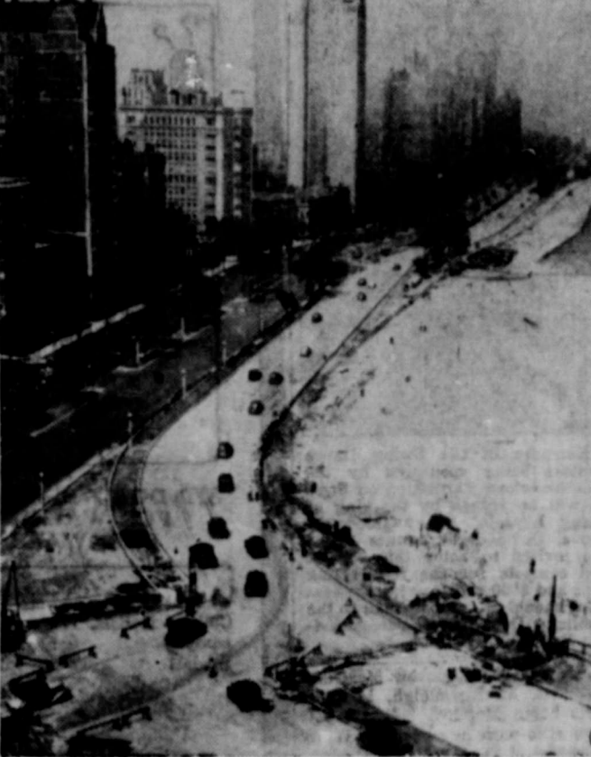
Stretching for miles along the lake front in the shadow of the city's skyscrapers, Chicago's new Lake Shore drive speedway is pictured above. Just inside the new roadway is the old drive, now relegated to slower and heavier vehicles.
