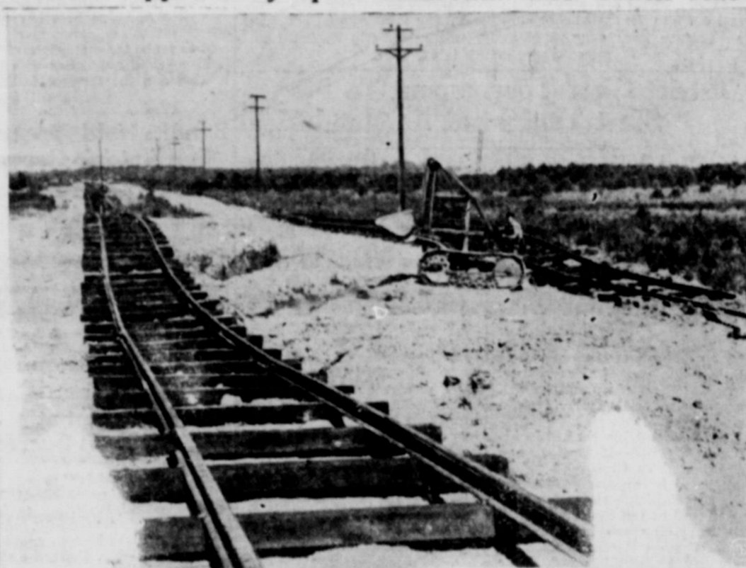
So flimsy that a freight train probably could not pass over the rails without disaster, two railroads raced to complete spurs across the New Jersey meadows to tap the lucrative freight business of the huge new automobile assembly plant at Linden, N. J. The hasty construction, which did not attempt a permanent roadbed, was undertaken to establish priority for right of way. Paralleling each other above are the Pennsylvania, left, and New Jersey Central spurs.
