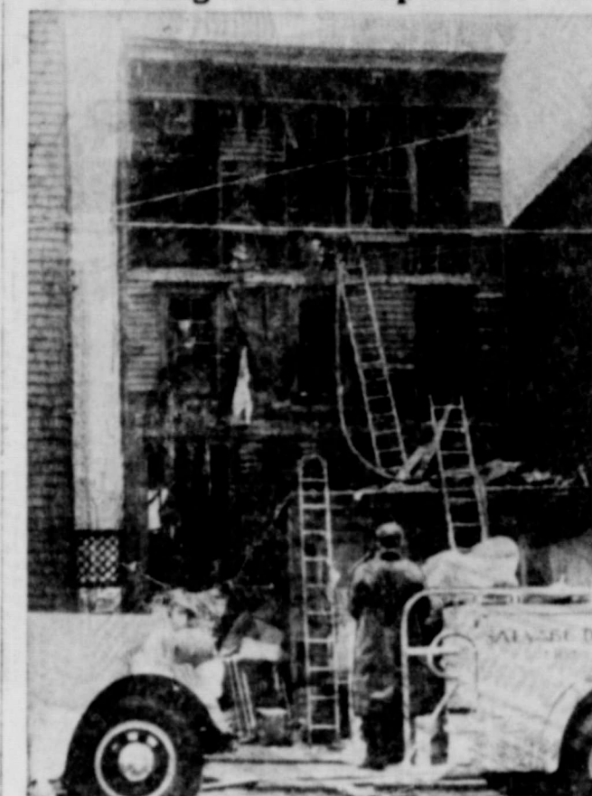
Flames fed by junk stored on the ground floor created an inferno that trapped and burned to death seven members of Mrs. Rose Burkhardt's family, including five children, at Jersey City, N. J. Pictured is the charred skeleton of the frame building in which they lived.
