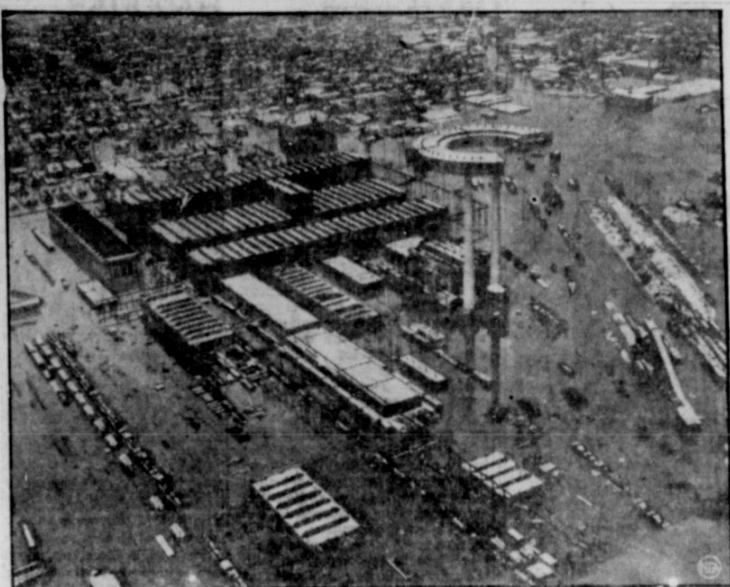
Evacuation of Paducah's 33,500 inhabitants had just been ordered when the above air picture of the flooded Kentucky town was taken. Shown slightly at the left is the Paducah power plant, disabled by the lapping waters which crept over the ground floor. Notice the inundated railroad tracks and how the flood waters extend almost completely over the business and residential sections. The Kentucky river was reported at the highest stage in history.
