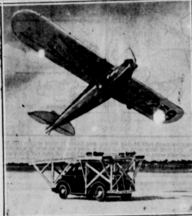
It looks like a stunt, but it may be a common sight at airports throughout the country if low-powered planes come into general use. One handicap of economy planes has been inability to develop speed enough in a short run to raise the ship off the ground. At Miami, Fla., Mike Murphy did it this way—zooming into the air from the top of a speeding auto on which a take-off platform had been built.
