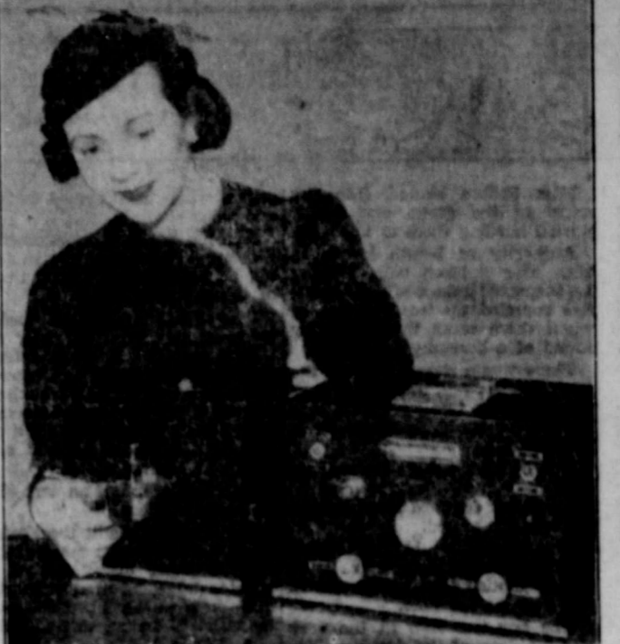
Loretta Poynton, NBC radio star, stands aside while her wrist watch performs before a special microphone for watches, which is part of a new time saving, time testing machine developed by Montgomery Ward engineers to cut days from the time required to test a watch for accuracy. The special microphone transmits the watch's ticks to a chart and tells in 15 seconds just how slow or fast a watch is regulated in any one position, an operation which formerly required days. The company has just installed these machines in all of its watch shops where all watches are scientifically tested before being sent out.
