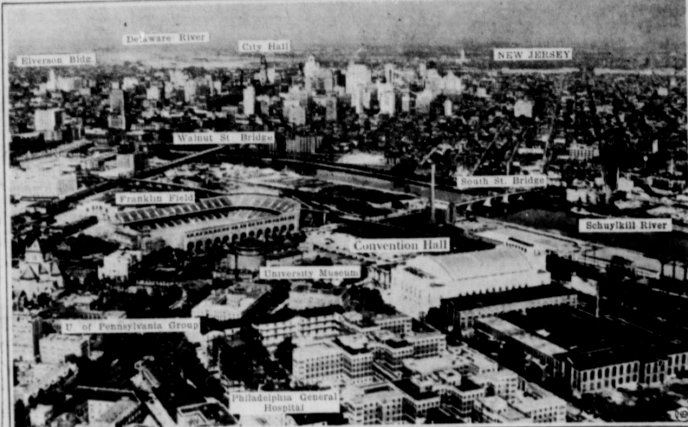
In the section of Philadelphia pictured in this graphic airview, the nation's outstanding Democrats will gather, in June, to renominate President Roosevelt. Center of activity then will be the convention hall shown at lower right. Buildings in the foreground, at left, are the University of Pennsylvania group. Nestling in the cluster of skyscrapers shown in the distance, beyond the Schuylkill river, are such historical landmarks as Independence Hall, "the birthplace of American liberty"; 209-year-old Christ Church, in which President Washington worshiped; Betsy Ross' house, where the first Continental Congress met in 1774. Other points of interest are indicated above.
