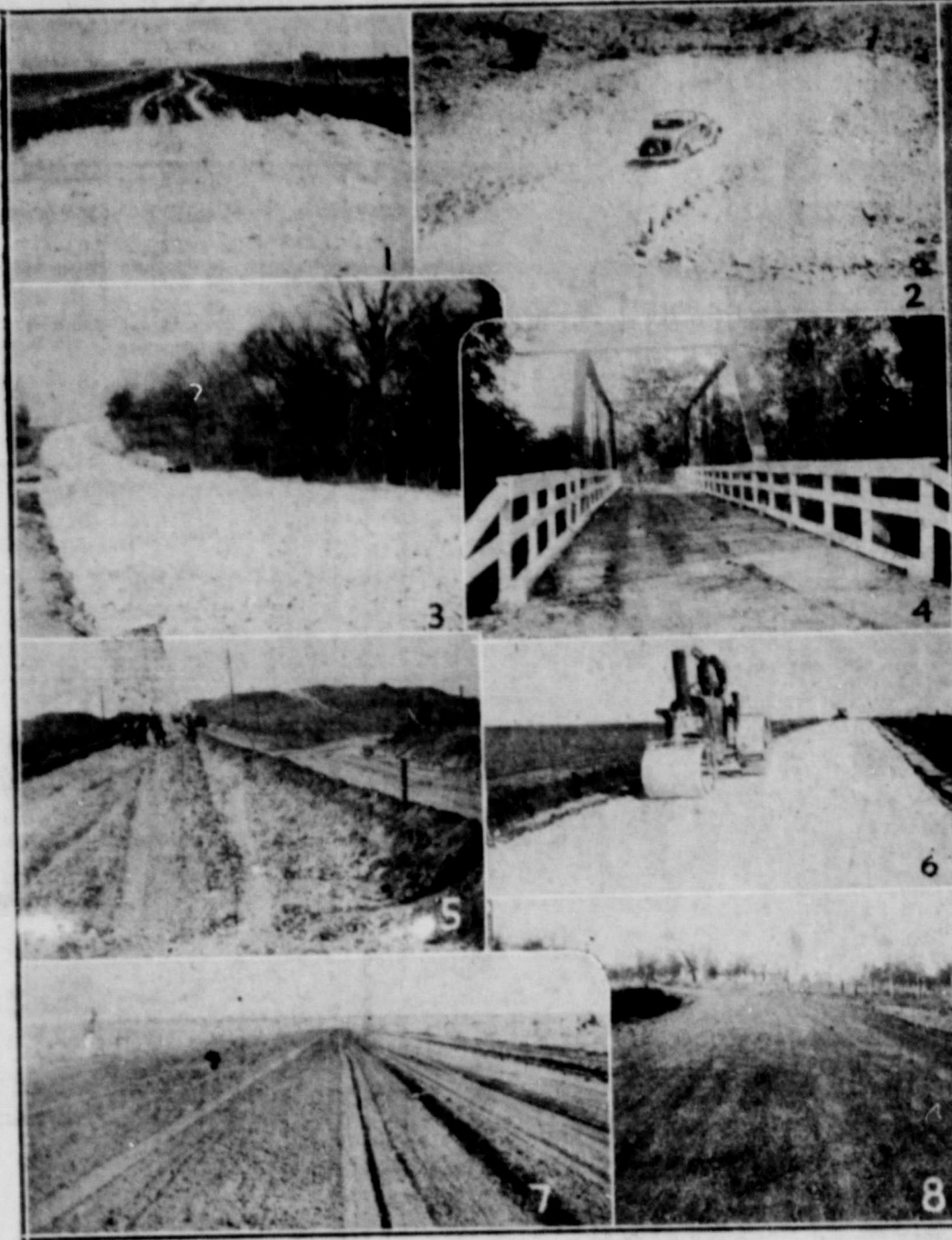
Here are glimpses of various stages of work on the 7,000 miles of farm-to-market roads being built and improved by Works Progress Administration workmen in Texas. Showing views of lateral roads in every stage, from unimproved and virtually impassable routes to smooth all-weather completed roads, the above scenes include: (1) An Ellis county road, showing the project partially completed, contrasting the weather-proof sledged stone surface course with the black unimproved road which was almost untraversable in wet weather. (2) View of Hair Pin Curve at south end of Quitman Canyon. Forty-three miles of road is being improved along this Hudspeth county route. (3) Stone topping awaiting crusher on the Dowdy-Ferry road in Dallas county. (4) Here is a completed bridge, one of the 21 such structures being rebuilt or repaired after flood damage in Navarro county. (5) Men spreading caliche for an all-weather surface on the Miami-Pampa road in Roberts county. (6) An all-weather road between Ovilla and Midlothian being smoothed in Ellis county. This route goes through rich farming country and will facilitate transportation of farm products. (7) A straight wide road bisecting farm lands near Abernathy in Hale county. (8) This completed smooth gravel road leads from Gilmer to Big Sandy in Upshur county.
