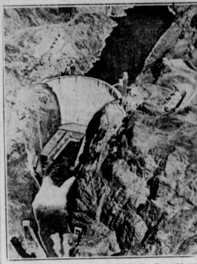
Not a tiny model, but the real, massive Boulder Dam, with great torrents gushing through its spillways for the first time, is pictured in this striking view, taken from a plane high above the earth. Enough water to float a battleship poured from Boulder Lake through the intake towers, shown behind the dam, and out the giant spillways, so government engineers could test the equipment.
