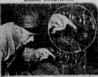
Workman indicating five-cent piece balanced on its edge on the cylinder head of a Hudson engine rotating at 2, 200 revolutions per minute.
