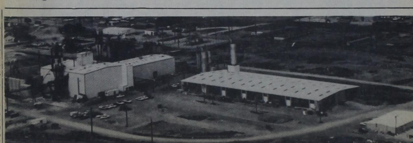
BIRD'S EYE VIEW of Dimmitt Agri Industries' completed corn wet-milling plant from a southwest angle shows the millhouse and refinery (left), with a feeder line coming from the cooperative's elevators, which are to left of the photo. The large, low building in center is the warehouse-workshop, and the smaller building at right is the former Catholic Community Center, which has been converted to
