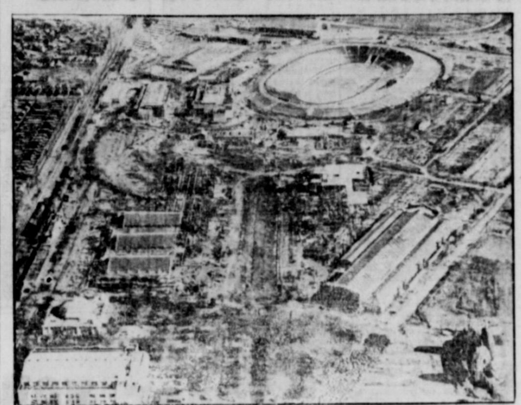
Five thousand men are laboring on three eight-hour shifts to complete construction work by June 6 on the Texas Centennial exposition grounds, at Dallas, shown in aerial view above. In the left foreground is the administration building, first to be completed. From that structure to the race tracks, just visible beyond the stadium, the distance is one mile. In the right foreground is the state fair auditorium.
