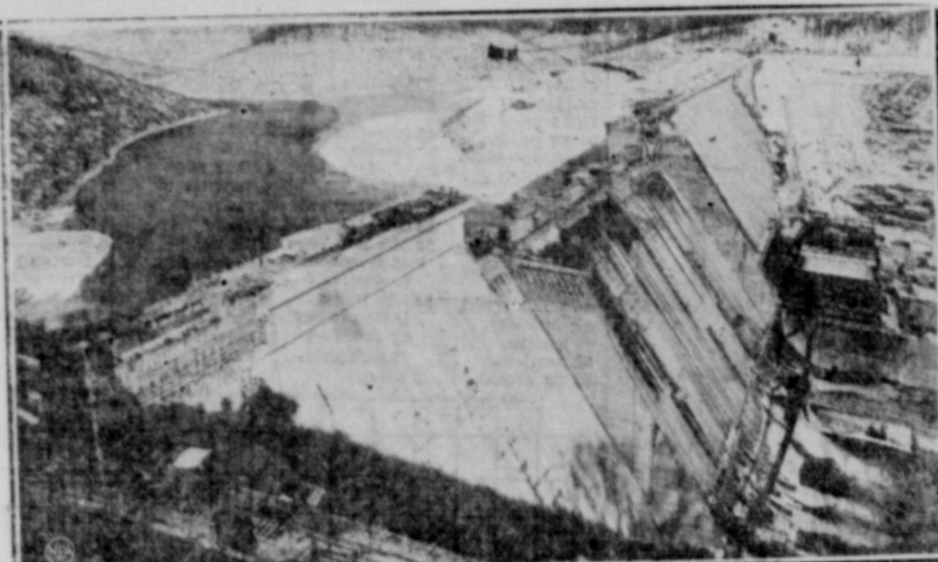
A mighty barrier 253 feet high and 1900 feet long, Norris dam, as pictured here, stood virtually completed as the U. S. Supreme Court decided on its ruling on validity of the giant TVA project, of which the dam is a major unit. With exception of the spillway gates, the concrete roadway across the top, and the powerhouse, work will be finished within a month, as all but 10,000 of the 1,000,000 yards of concrete has been poured. The $24,000,000 structure, on the Clinch river in East Tennessee, will back water up for 80 miles, forming a lake with an 800-mile shore line.
