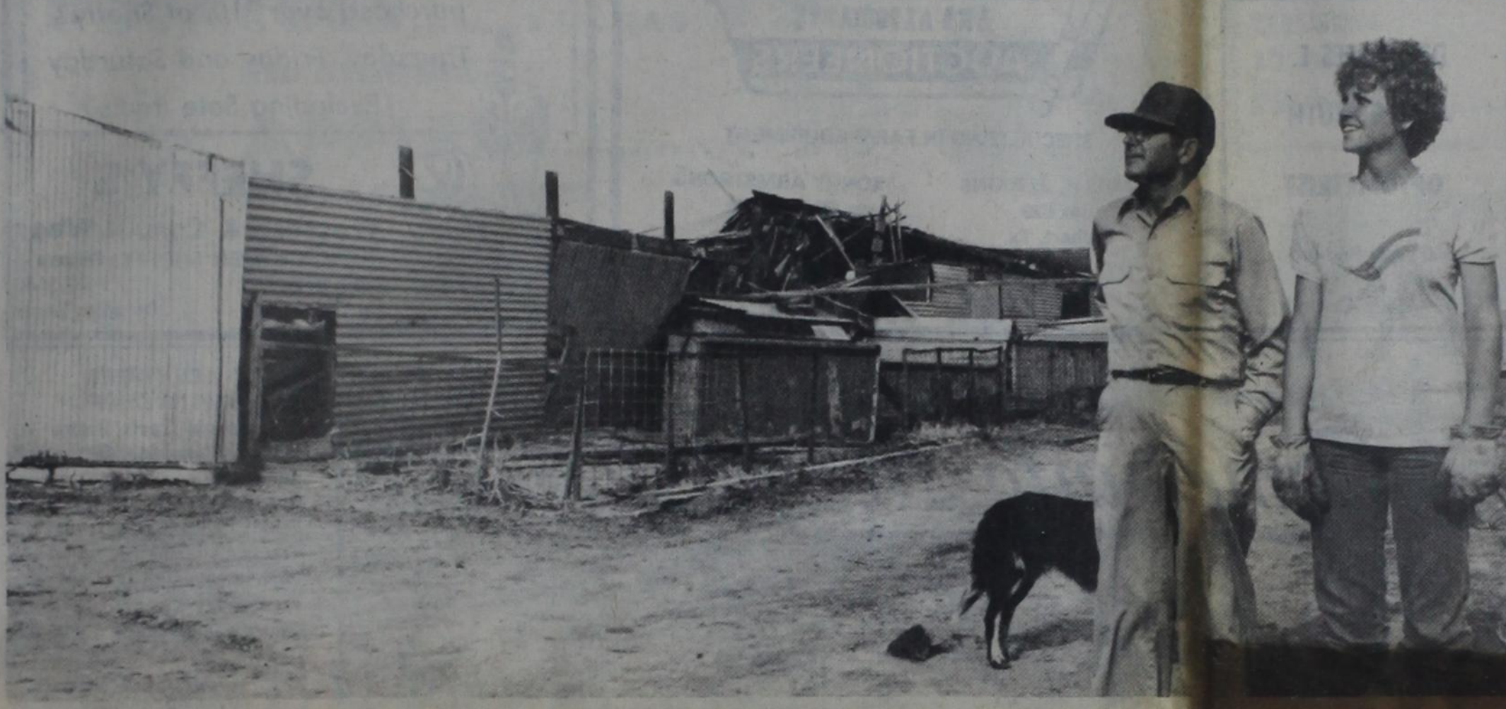
SURVEYING THE DAMAGE —Wade Mills and his granddaughter-in-law, Tammy Robb, look over the damage caused by a tornado on the Mills farm between Hart and Nazareth late Monday night. In background is what's left of a large hog-nursery barn after the tornado had ripped off its roof and some of its walls. In the direction that Mills and Mrs. Robb are looking, a quonset barn was ruptured and two cotton strippers and a Grain Kart were blown over.
