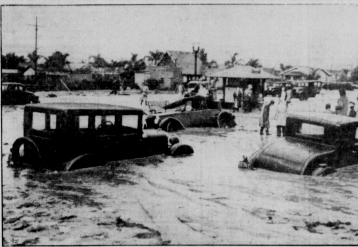
Half-buried in a sea of mud, automobiles dotted the scene of devastation after raging torrents, bearing tons of silt and rocks, swept over Los Angeles county, Calif., killing more than 40 and causing $5,000,000 damage. The view here is in Glendale, a suburb of Los Angeles, with booted men and curious women inspecting the ruin and barefoot children enjoying a mud wade.
