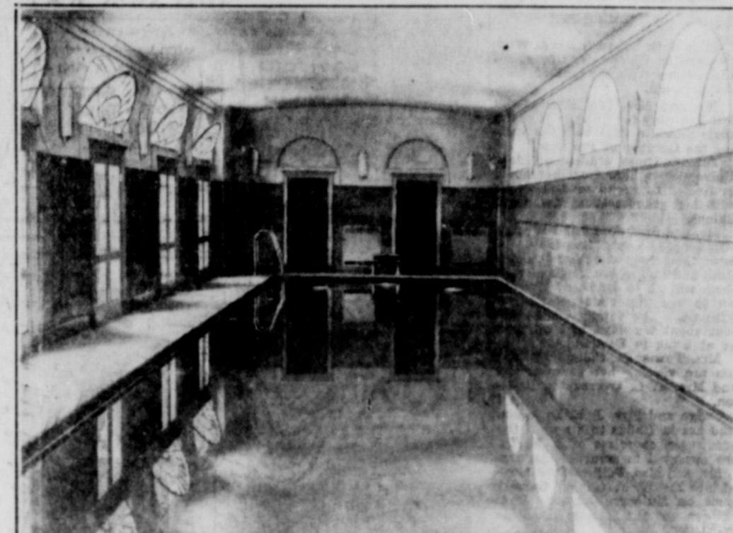
Here is the White House swimming pool, ready for the presidential plunge. Built with funds collected by popular subscription, the pool ranges from four to eight feet in depth.
