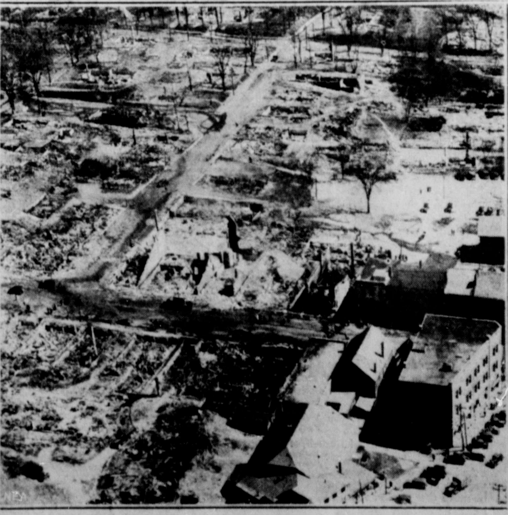
Here is a graphic aerial view showing the devastation caused by the $3,000,000 fire that swept Ellsworth, Me., for seven hours, destroying 200 dwellings and business houses, and rendering 400 homeless.
