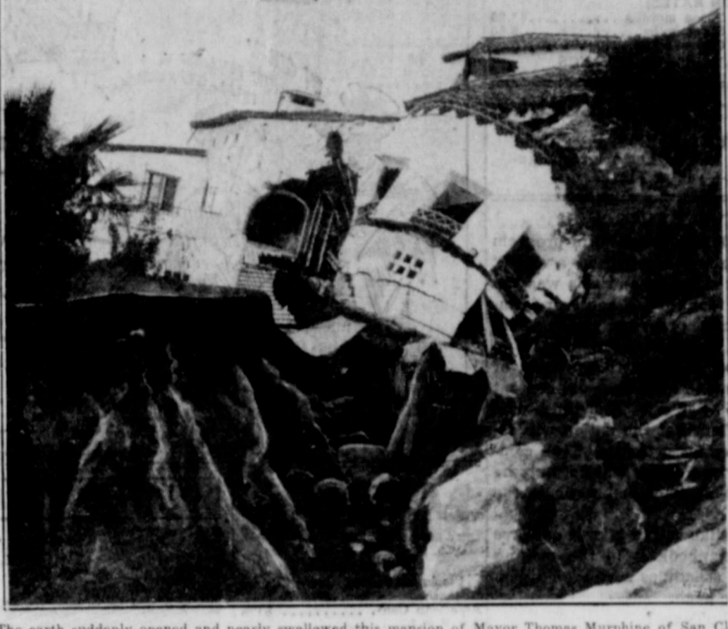
The earth suddenly opened and nearly swallowed this mansion of Mayor Thomas Murphine of San Clemente, Calif. The wrecked mountain home lies in a fissure 60 feet wide and 50 feet deep. The cavern in the foreground was a spacious lawn. A landslide nearly preceded the earth's separation.
