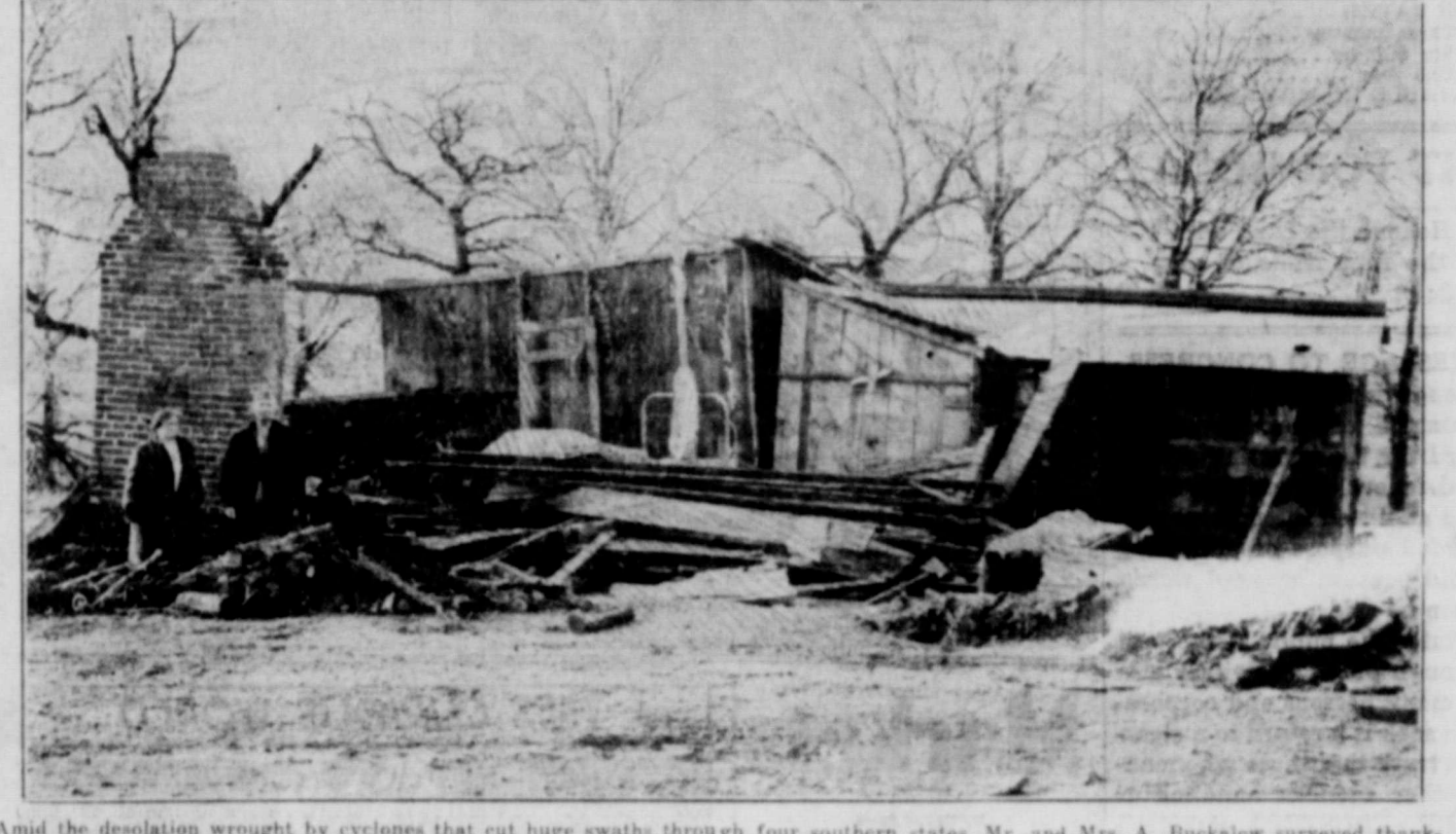
Amid the desolation wrought by cyclones that cut huge swaths through southern states, Mr. and Mrs. A. Buckalew surveyed thankfully the wreckage of their home near Mount Sylvania, Smith county, Texas. The couple and three children escaped unhurt when the frame structure crumpled in the cyclonic fury, that killed two persons near by and took a toll of 68 deaths in Texas, Arkansas, Mississippi and Louisiana.
