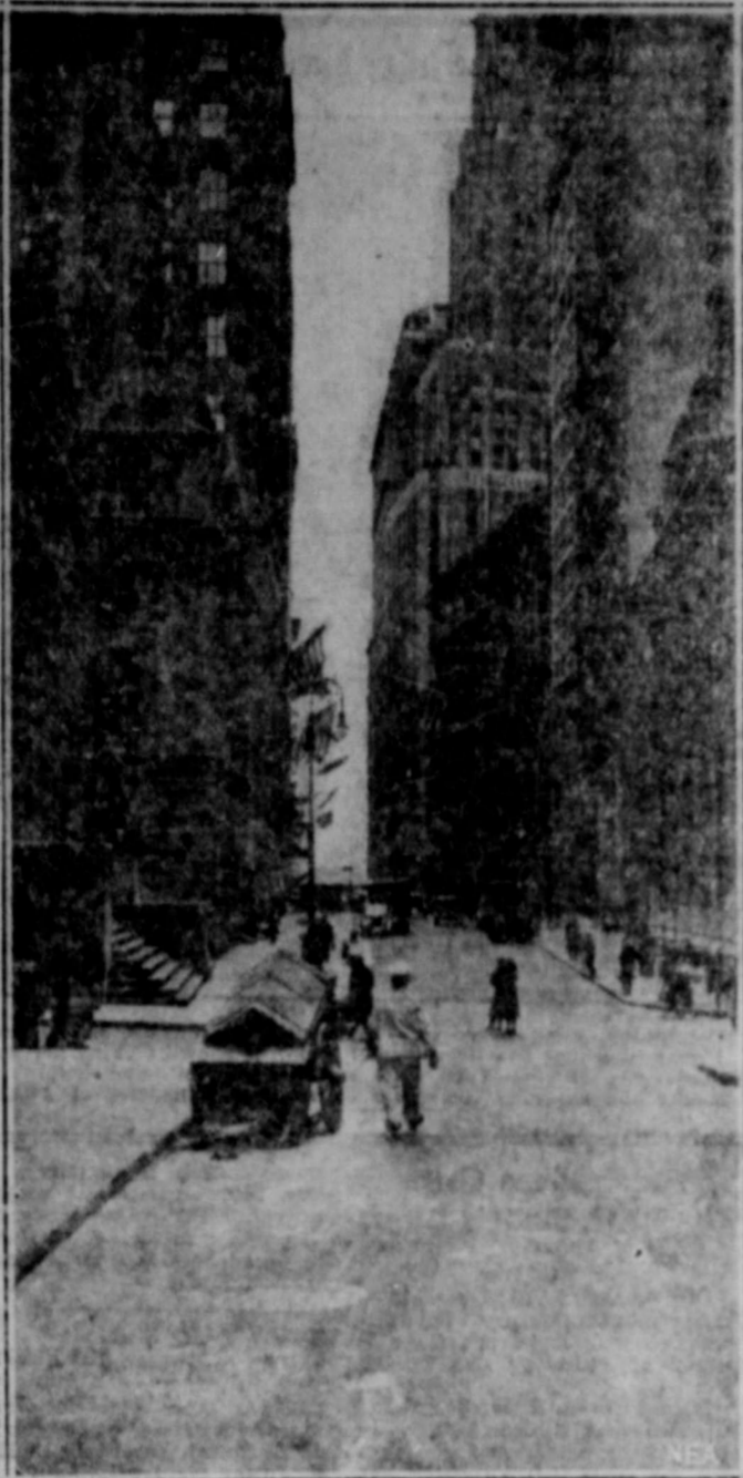
World-famous Wall Street's narrow pavements as they appeared, comparatively deserted, at the start of the banking holidays in New York. At extreme left: the sub-treasury building; the statue of George Washington surveys the unfamiliar scene. At extreme right: the House of Morgan; symbolic of high finance.
