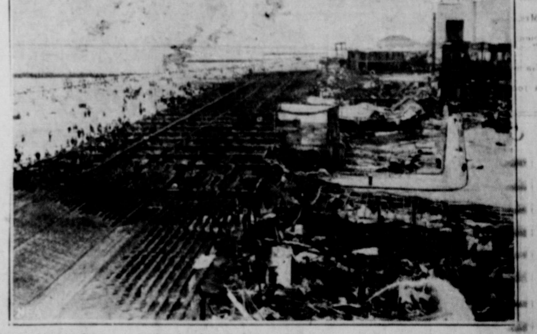
The fire-blackened framework of Coney Island's famous boardwalk and the charred ruins of adjacent buildings are shown in this graphic photo taken after wind-driven flames had lapped up water-front property valued at $5,000,000. The blaze had hardly been quenched when thousands of New Yorkers returned to the beach (as seen at the left) to escape the city's mid-summer heat. Hundreds were left homeless by the spectacular fire that ravaged four square blocks.
