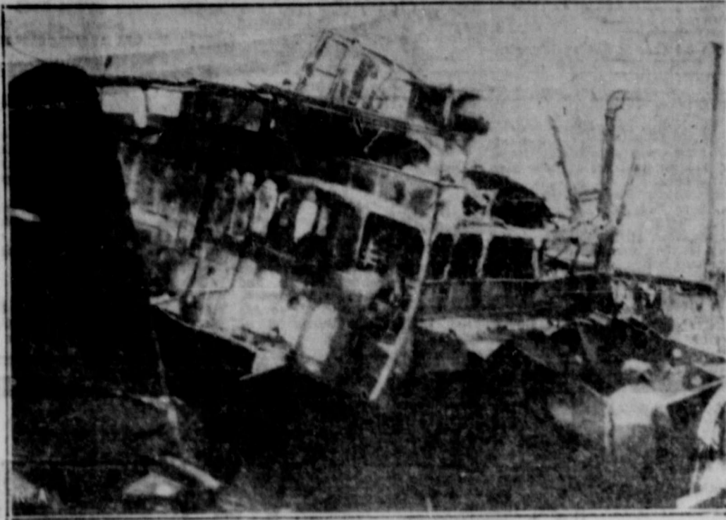
Four explosions and an intense fire on the Tanker Bidwell as she lay at dock in Marcus Hook, Pa., on the Delaware River, killed 17 members of the crew including the master, Captain Joseph Rivers, who died in his cabin attempting to save the logbook and papers.
