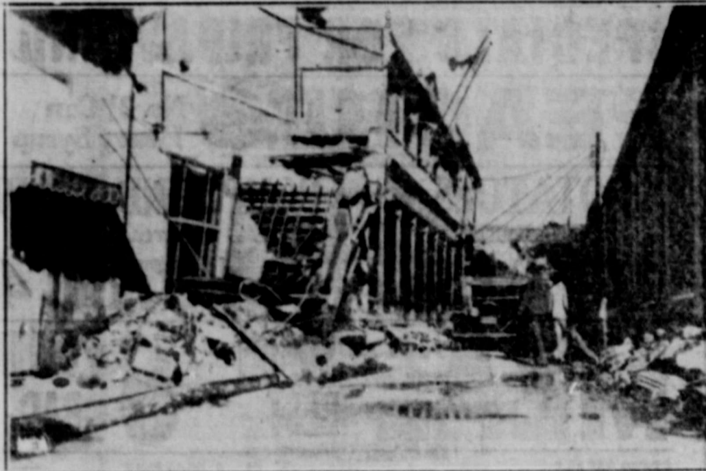
This picture, rushed by special plane from the scene to Atlanta, Ga., and telephoned from there for NEA Service, shows the damage done to buildings on one of the main streets of Santiago, Cuba, by an earthquake.
