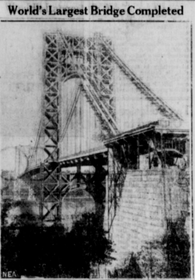
World's Largest Bridge Completed Ready for use after four and a half years of record-breaking construction, the George Washington Bridge here is pictured as it now spans the Hudson River between upper Manhattan and northern New Jersey. The structure cost $400,000,000 and its central span is 3500 feet in length.
