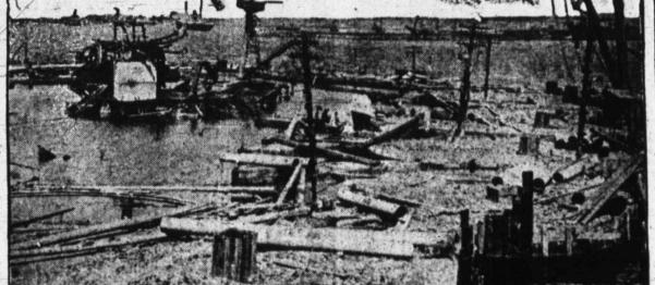
The raising of the Maine-Photograph showing the completed offerda ms built around the wrock of the surken battleshop in Havana Harbor. In the background can be seen the mast of the ill-fated ship. The cofferdams, some of which appear plainly in the foreground, have all been completed and filled in with cement and The work of pumping out the water has started, and already a tangled mass of wreckage has been uncov ered, which was hidden by the water since the vessel went down in 1898.
