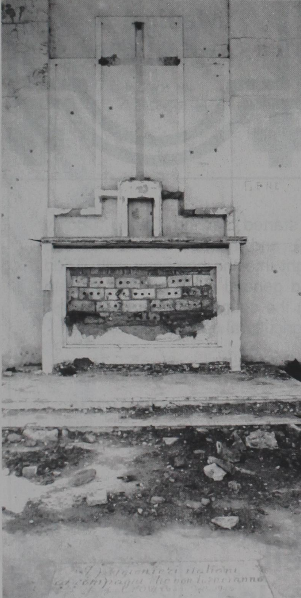
INSIDE THE CHAPEL, despite years of vandalism, one can see the meticulous craftsmanship that went into the construction of the memorial. The Italian prisoners worked their plaster for the walls and altar until it approached the smoothness of granite and marble. (Photo by Don Nelson)
