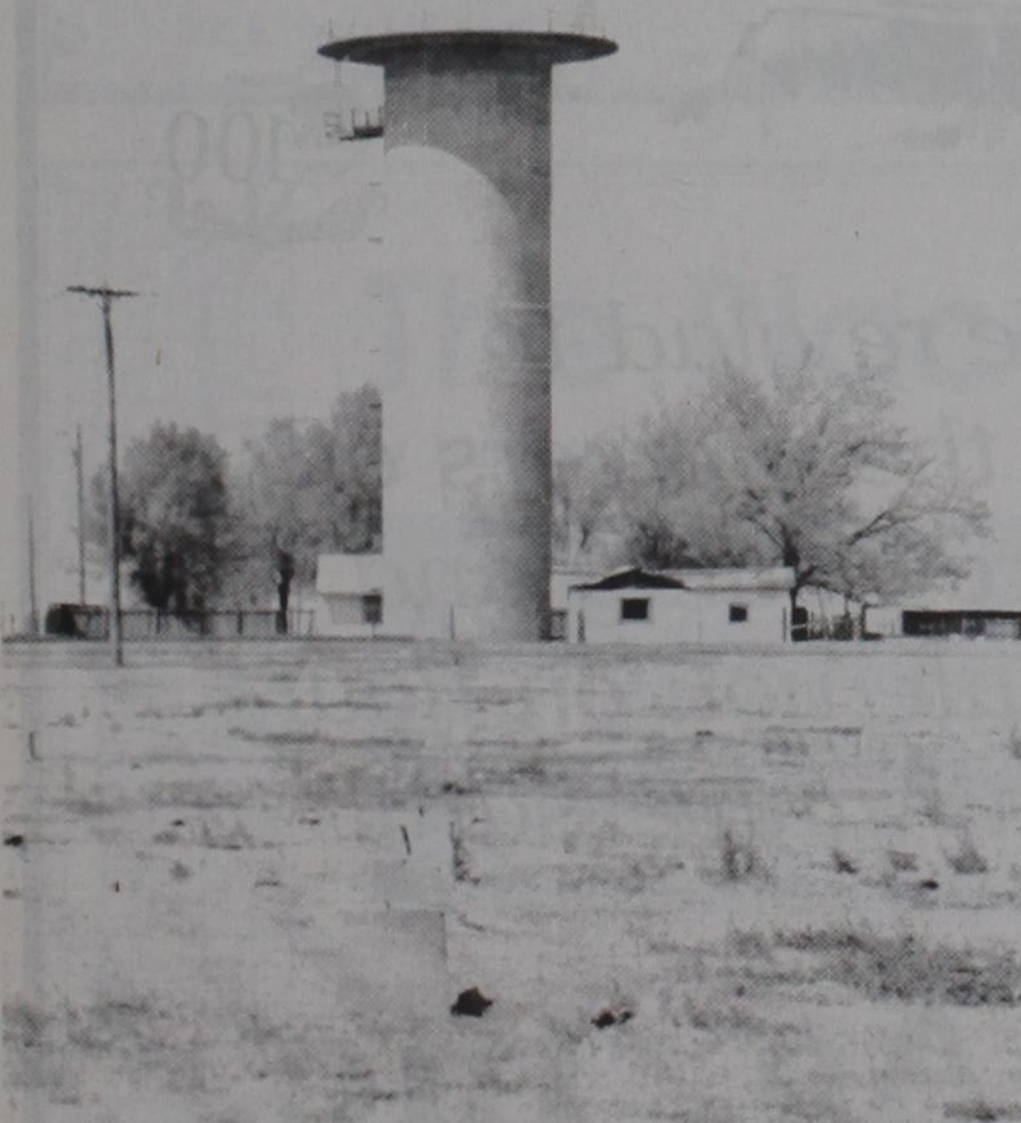
THE WATER TOWER'S concrete cylinder, minus its tank, stands as a lone sentinel over the other remnants of the Hereford POW Camp. The tower's wooden ladder is still intact, although the screening for the ladder's safety tunnel is gone. The tower is now unsafe to climb. Rising out of the native grass in foreground are the concrete piers, sunk four feet into the ground, which supported many of the camp's buildings.
