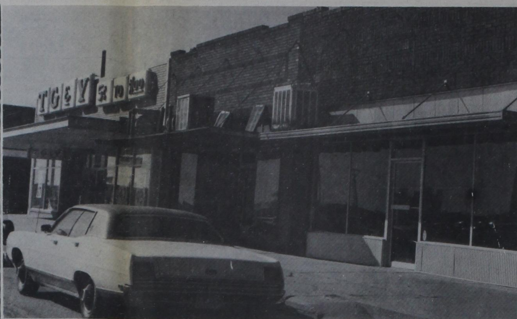
ALL THIS SPACE WILL BECOME ONE BIG T.G.&Y. STORE ... Two buildings on right will be torn out after first of the year
