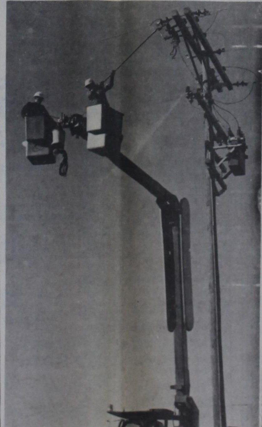
FINAL ELECTRICAL CIRCUIT RE-ESTABLISHED . . . By Public Service crew northeast of Dimmitt
