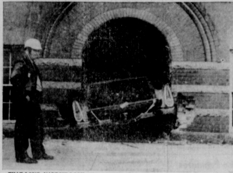
THAT LONG, NARROW LOOK—Slamming into the doorway at high speed, this station wagon has widened the entrance to a church in Petersburg, Va.
