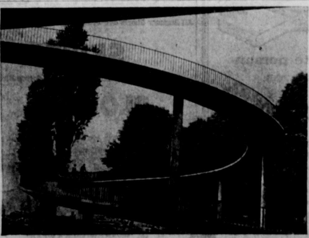
RAMBLING RAMP—Spiraling gracefully upward, this circular ramp was built especially for bicyclists and pedestrians at Dusseldorf, West Germany. Much easier to ascend with a bike than the traditional stairs, the ramp leads to the lofty Dusseldorf Rhine Bridge.
