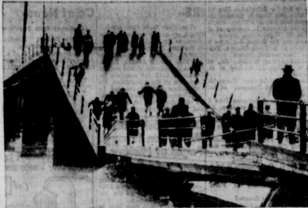
TWO-LEVEL BRIDGE —Pedestrians walk uphill as they cross this bridge in Concepcion, Chile, leveled by the great earthquake.
