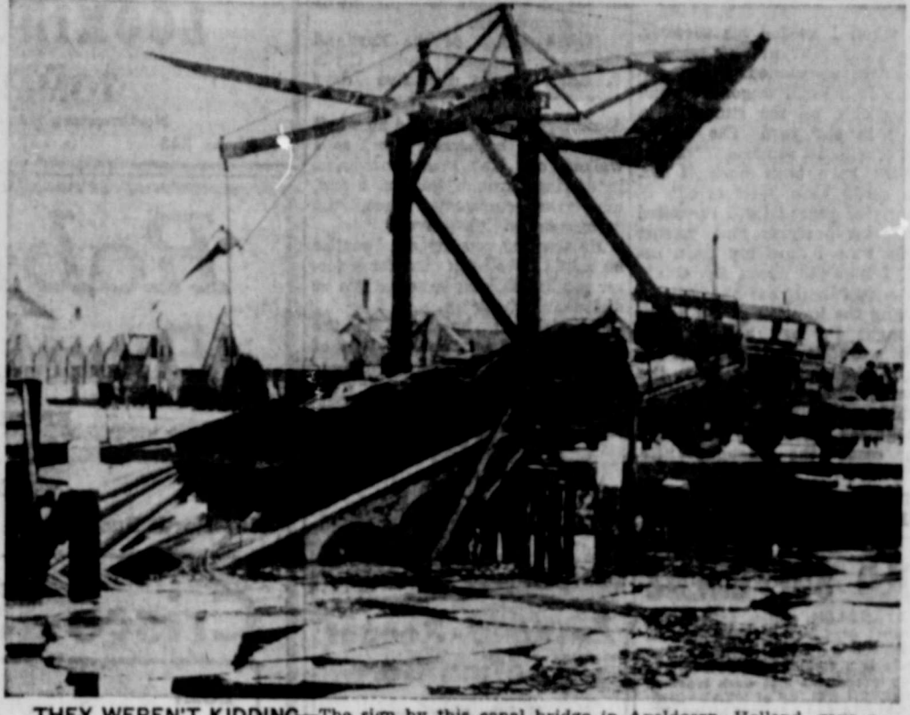
THEY WEREN'T KIDDING—The sign by this canal bridge in Apeldoorn, Holland, gave a maximum weight of one ton. The driver of this trailer truck loaded with 12 tons of iron pipe perhaps thought—like motorists everywhere—that sign makers are just alarmists. But they weren't kidding.
