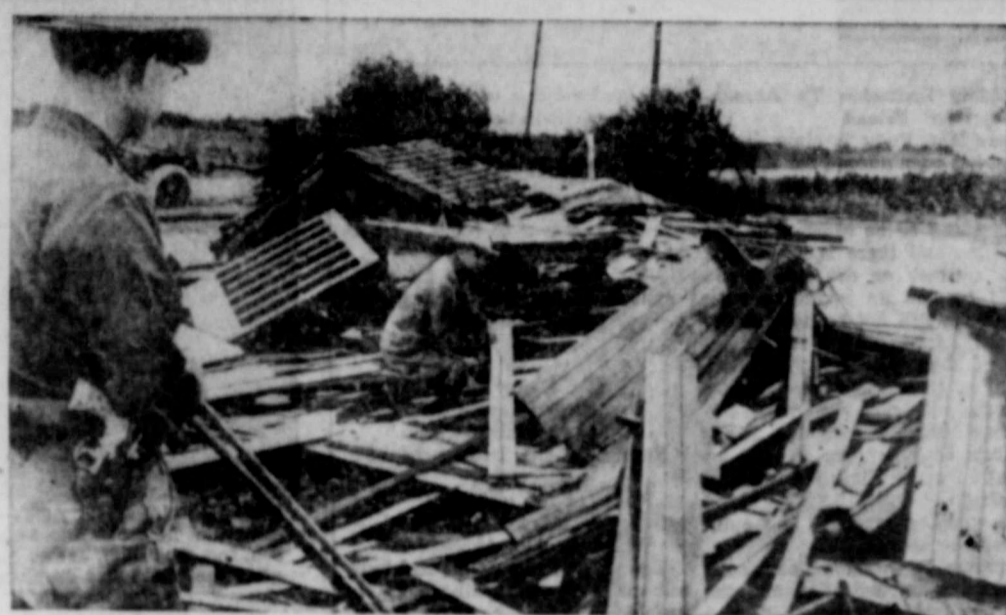
ALL THAT'S LEFT—Little more than kindling wood remains of a Baptist church after a tornado churned through New Mesquite, Tex. Nobody was killed when the church collapsed.
