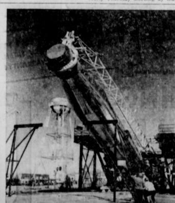
MUSCLED MISSILE-Pictured, above, at San Diego, Calif., is a new erector-launcher for the Atlas intercontinental ballistic missile, shown. Designed by the manufacturer who assembles the Atlas, the huge boom has the launching mechanism at its base. Use of the sprawling mechanism permits horizontal
