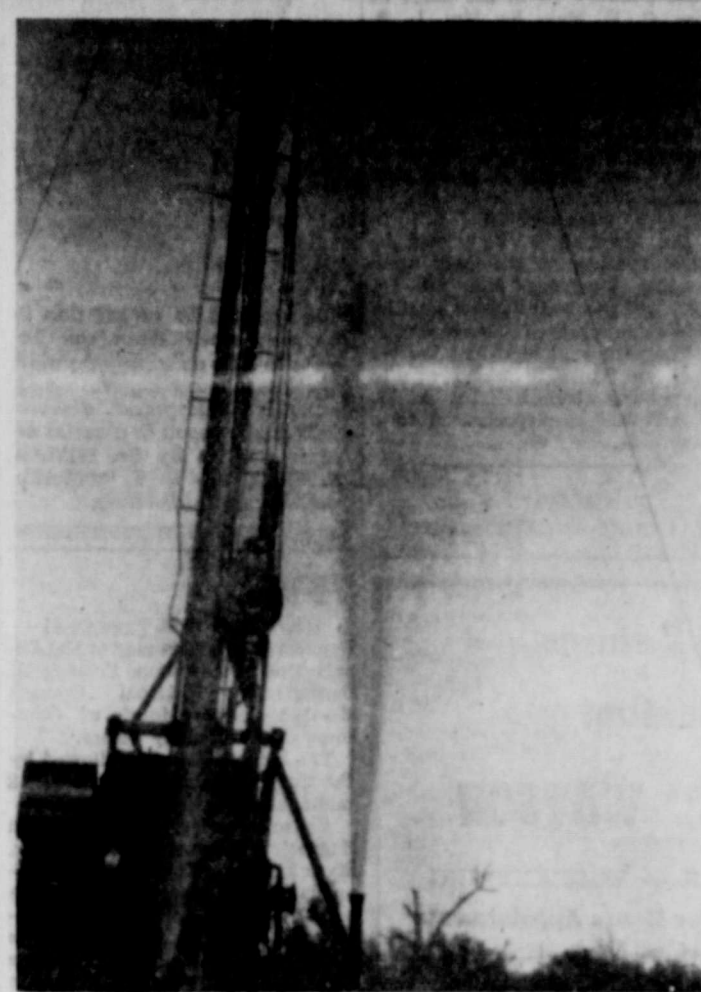
FLOWING OIL—Here oil flows from a well, at a total depth of 1,800 feet, located 12 miles northwest of Ranger. More wells are expected to be drilled in the area. This wildcat is producing about two barrels an hour.
