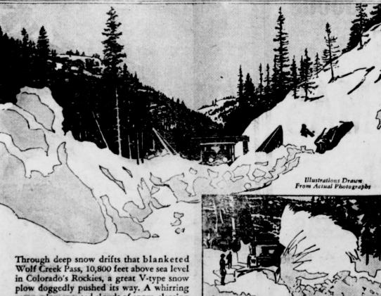
Through deep snow drifts that blanketed Wolf Creek Pass, 10,800 feet above sea level in Colorado's Rockies, a great V-type snow plow doggedly pushed its way. A whirring rotary plow spouted clouds of snow, clearing the roadway. And soon, despite temperatures drifts below zero workers of Liberty. tures daily below zero, workers of Liberty Truck & Parts Co., of Denver, had opened the 15-mile road.
