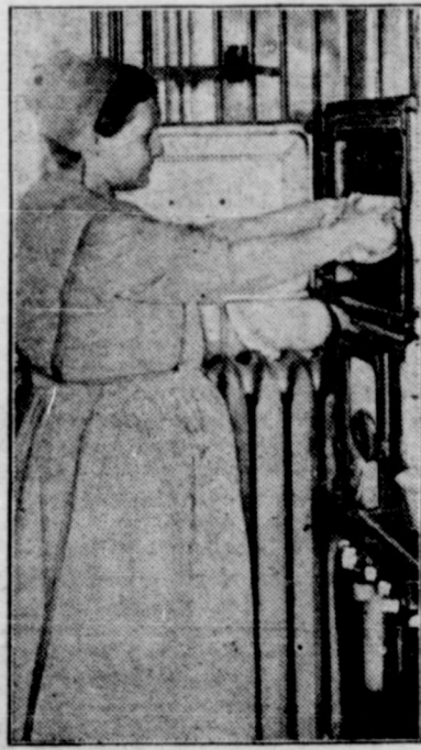
Pennsylvania Farm Kitchen Electrically Equipped.
