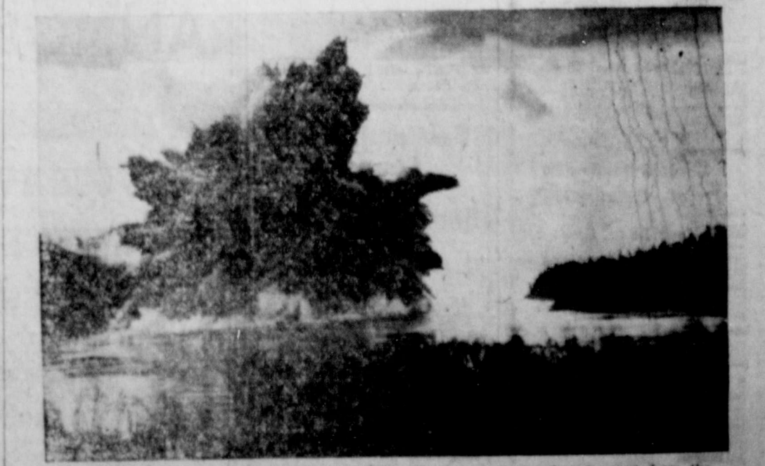
DREADED MARINE HAZARD DESTROYED—Water and shattered rock erupt from the effects of 1,375 tons of explosive, one of the largest, non-nuclear blasts in history. The Canadian Department of Public Works set off the explosion to level Ripple Rock, an underwater hazard in British Columbia's Campbell River that has claimed over 100 lives and destroyed about 170 ships in the past 100 years. The three-million-dollar project was designed to shatter about 373,000 tons of rock. Wavy lines at right are from rockets fired by scientists testing the explosion's force.
