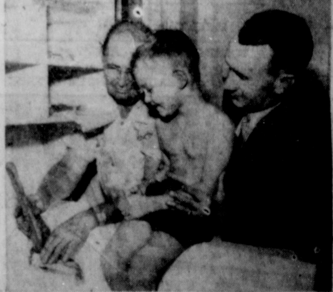
DALE REESE—five-year-old Sherman boy smiles his approval as a workman installs a new raised bathtub completing a $26,500 remodeling program at the Texas Scottish Rite hospital for Crippled Children at Dallas. John McKee, right, hospital president, announced that the needed improvements were made possible by a recent grant from the Ford Foundation.
