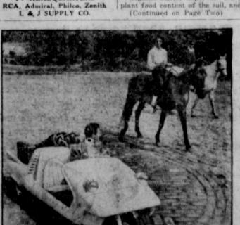
CET A HORSE-Riders in New York City's Central Park give the horse laugh to the driver of a three-wheeled utility car. Named the "Star," the tiny vehicle has a streamlined body of molded fiberglas and a one-cylinder German J.L.O. engine. The car has a maximum speed of 70 miles per hour, and is said to get 80 miles to the gallon. Less than three feet high, the Star is 10 feet, five inches long, 50 inches wide, and weighs only 400 pounds. The vehicle was designed for Basson Industries Corp.
