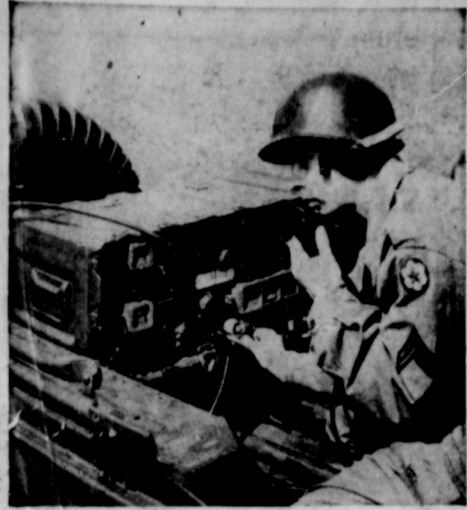
VOICE OF COMMAND —Corporal Albion D. Parsons, Hampstead, Md., talks to headquarters over the Army's powerful new long-range radio. Installed in jeeps, tanks or reconnaissance cars the radio—four times more powerful than the standard World War II model—has a range of up to 2,000 miles and can also be used to send or receive messages at 100 words a minute on teletype.
