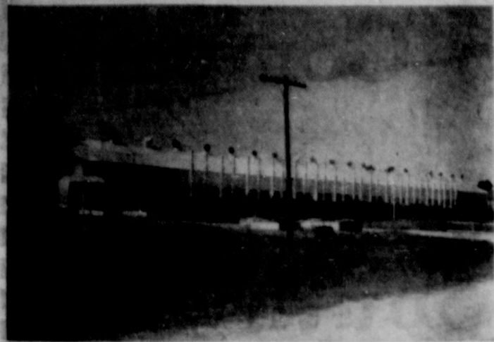
Lone Star Compressor Station No. 3
