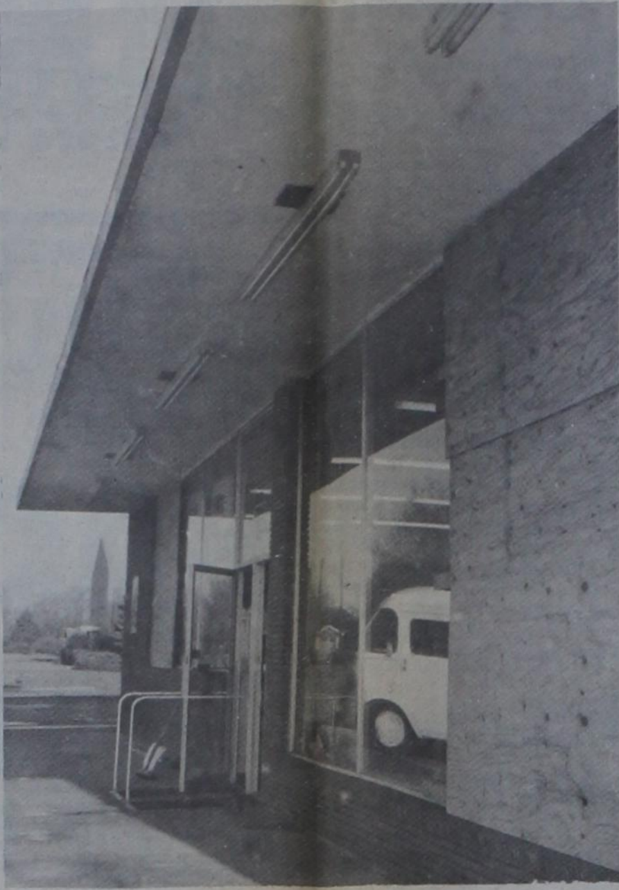
PLYWOOD WINDOWS AT DIMMITT SUPER MARKET ... Owner Walt Hansen knew they were going, and waited
