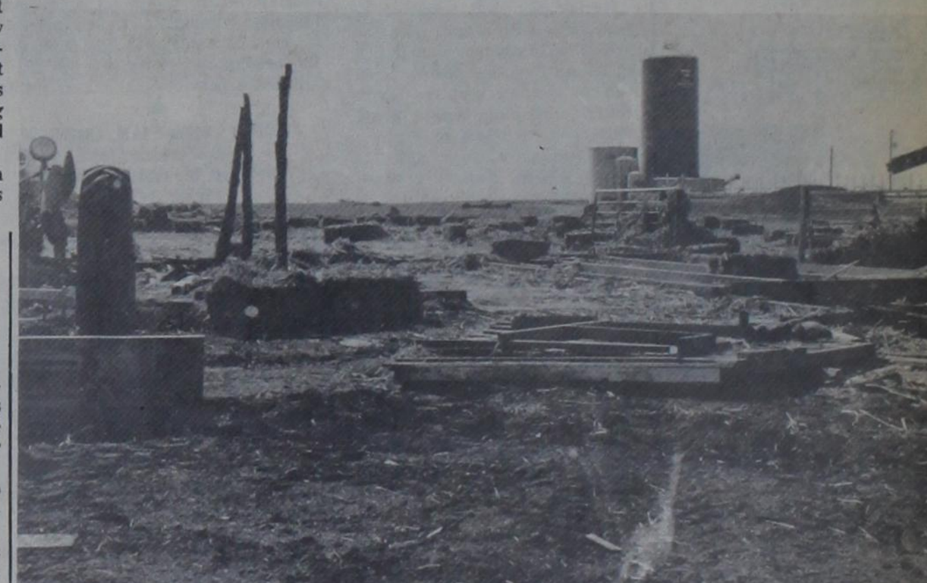
TORNADO HURLED HAY BALES OVER BAGWELL FEED LOTS ... West wall of storage barn lies in foreground
