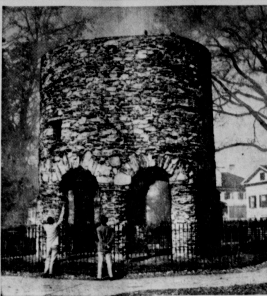
EARLIEST CHURCH — MAYBE . . . Excavation of this stone structure at Newport, R. I., may prove it to be the earliest Christian church in the western hemisphere. Research now is being undertaken by the Preservation Society of Newport to investigate the claim that it was built by Norsemen more than 100 years before the arrival of Columbus. Counter contention is that structure is simply an old windmill built in the 1660s by Benedict Arnold, then governor of Rhode Island.
