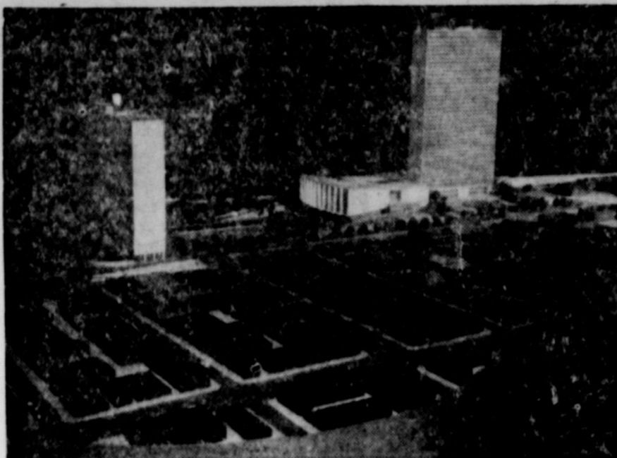
WORLD CAPITAL — CITY OF GLASS . . . Glass will be the main motif of the projected United Nations buildings in New York, shown here in a model. Most startling innovation is the use of double-paned glass sheets which provide for about a foot of space between inner and outer windows so that solar heat can be isolated, making it simple to keep buildings cool in summer. Coolness will be a vital prerequisite of any building housing some of the hot U. N. debates.
