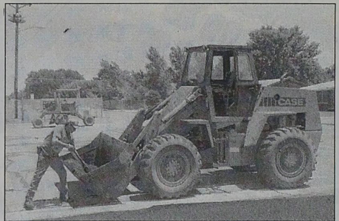
Johnny Rodriguez works on the parking lot at Richardson Elementary.
