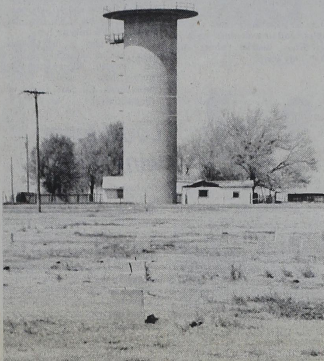
THE WATER TOWER'S concrete cylinder, minus its tank, stands as a lone sentinel over the other remnants of the Hereford POW Camp. The tower's wooden ladder is still intact, although the screening for the ladder's safety tunnel is gone. The tower is now unsafe to climb. Rising out of the native grass in foreground are the concrete piers, sunk four feet into the ground, which supported many of the camp's buildings. (Photo by Don Nelson)
