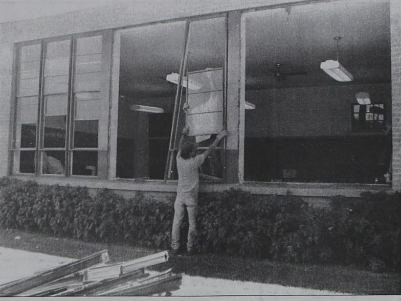
A STUDENT'S DREAM—They're not tearing up the school, just replacing the windows as part of the climate control improvement project at Dimmitt Middle School, which includes installation of air conditioning.
