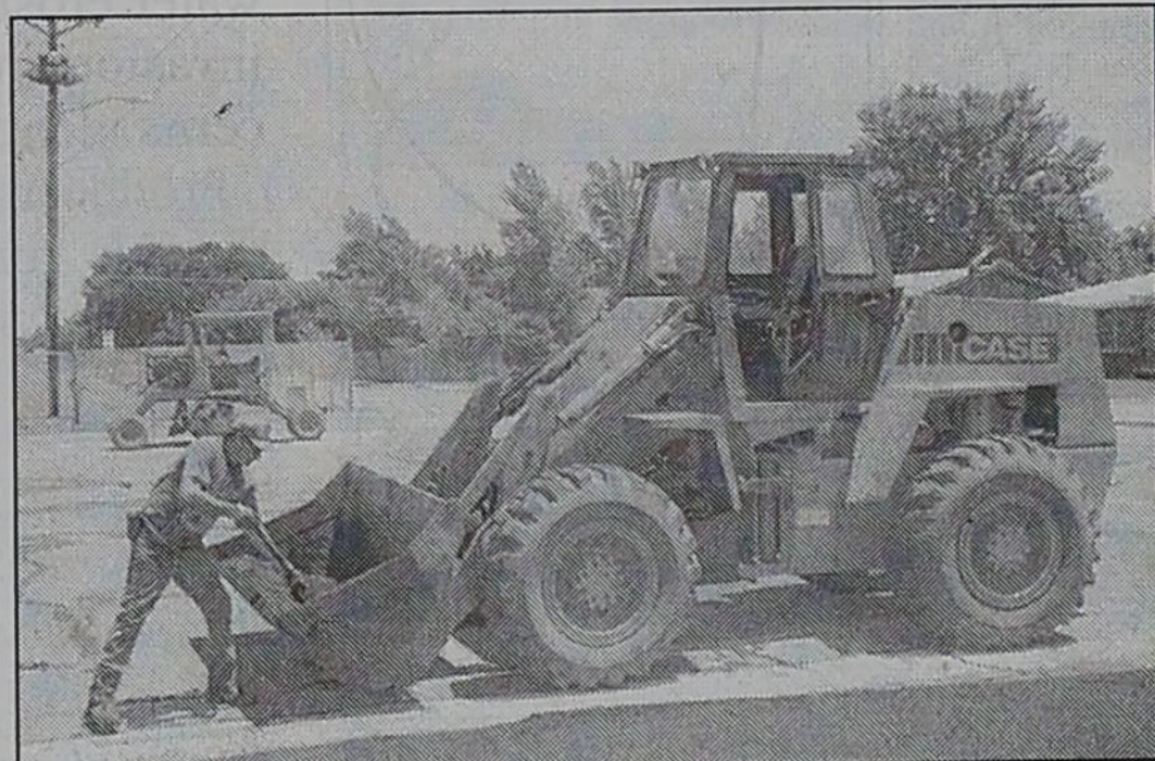
Johnny Rodriguez works on the parking lot at Richardson Elementary.
